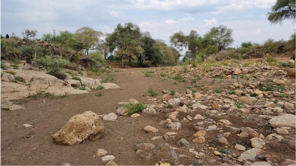
Figure 15. The river passage through the dyke. Rock can be seen on both the southern side (left in the picture) and northern side (right). The distance between the outcropping rock is approximately 30 m on the narrowest point
