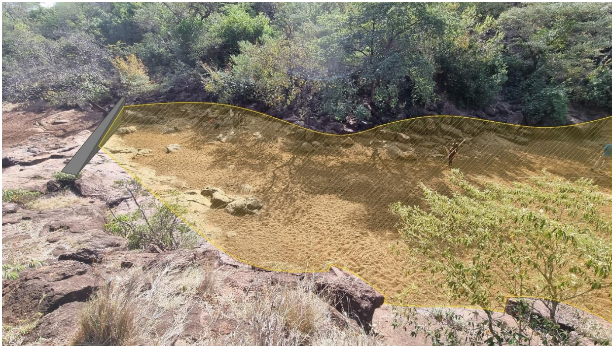
Figure 57. Conceptual sketch of the initial stage of a sand dam at the Kaloreng site (the dam height in the picture is around 1,5 m). Planned final total dam height is 3,5 m.
