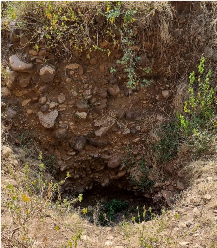
Figure 14. Water hole/dug well approximately 5 m deep.
